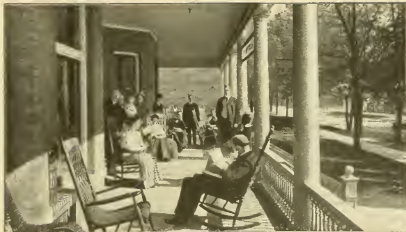
The Front Porch of The Glenwood
